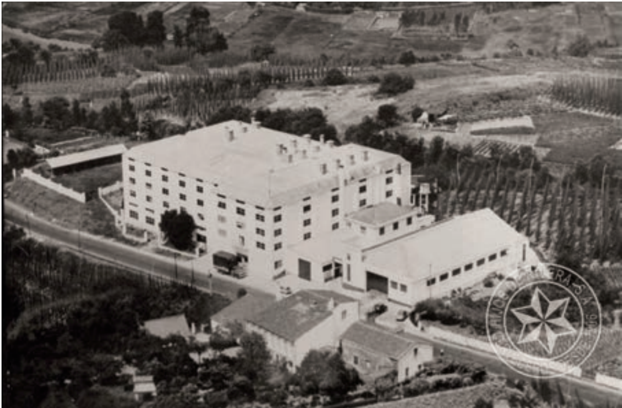
Figure 2. The hop processing plant in Betanzos near La Coruña.
